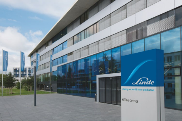
Linde GmbH, Linde Engineering, 82049 Pullach
